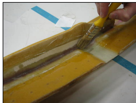
Figure 33: Smoothing the resin
